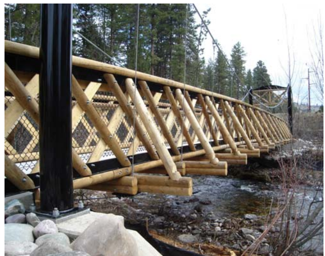
Figure 2. Cable suspension bridge across Rattlesnake Creek
