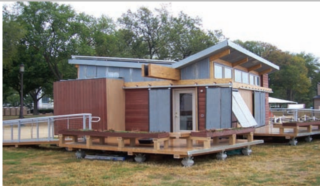
WSU solar decathlon house, on site in Washington DC, constructed with wood plastic composites fabricated at WMEL (2005)
